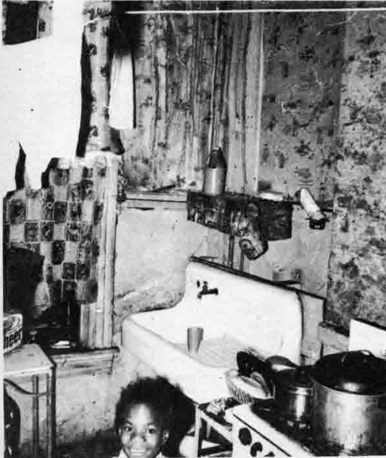
The ravages of lead poisoning are readily apparent in this inner city dwelling.
